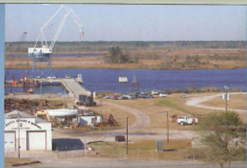
Shown here is the Carolina Marine Terminal site prior to construction. (Photo courtesy of Carolina Marine Terminal)
